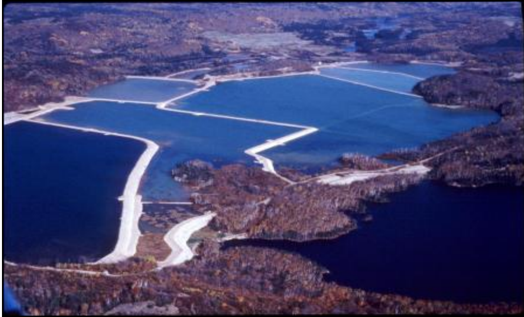
Photo 8: Control structures for engineered water cover treatment of acidic tailings.
