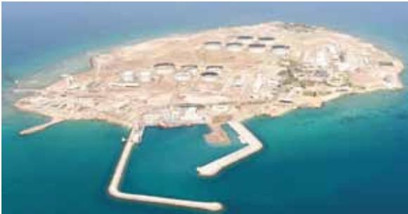
square kilometers, lies approximately 96 kilometers to the northeast of Doha. It boasts of 11 large crude oil storage tanks with a capacity of 5 million barrels. The island also encompasses pumping facilities, power generators,
